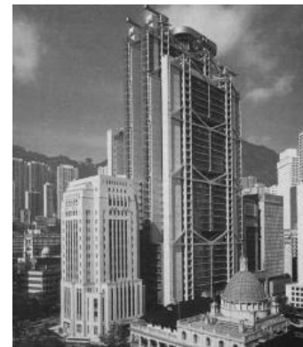
Figure 1 : The Hong Kong Bank building, designed by architect Norman Foster, features an exterior and interior structure that stands out prominently. This design directly contributes to the building's appearance. (Foster and Hunt.1998)
