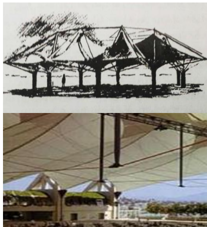
Picture 4: Sea World booth. (1980, San Diego, California; Structural Engineer: Horst Berger). Note that the compression bars used to maintain the vertical lines of the roof have eliminated the need for a central post. Additionally, the requirement for rope cables stretched under the perimeter structure has been removed, thanks to the horizontal restraint bars, which have resolved the issue of internal thrust forces. (16)
