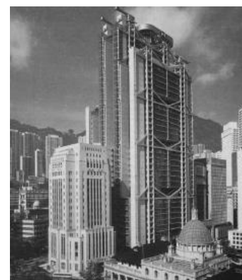
picture 1: The Hong Kong Bank building, designed by architect Norman Foster, features an exterior and interior structure that stands out prominently. This design directly contributes to the building's appearance. (Foster and Hunt, 1998)
