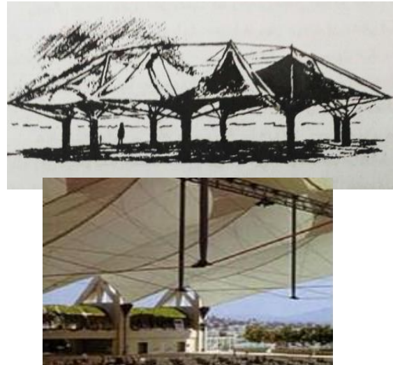
Picture 5: Sea World booth. (1980, San Diego, California; Structural Engineer: Horst Berger). Note that the compression bars used to maintain the vertical lines of the roof have eliminated the need for a central post. Additionally, the requirement for rope cables stretched under the perimeter structure has been removed, thanks to the horizontal restraint bars, which have resolved the issue of internal thrust forces. (21)
